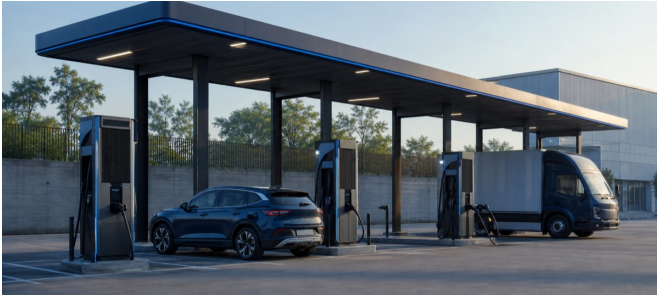
01 EV charging networks
